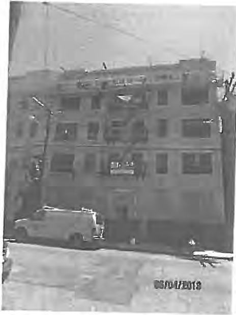
An exterior view of Bergen Court during the renovation project.
